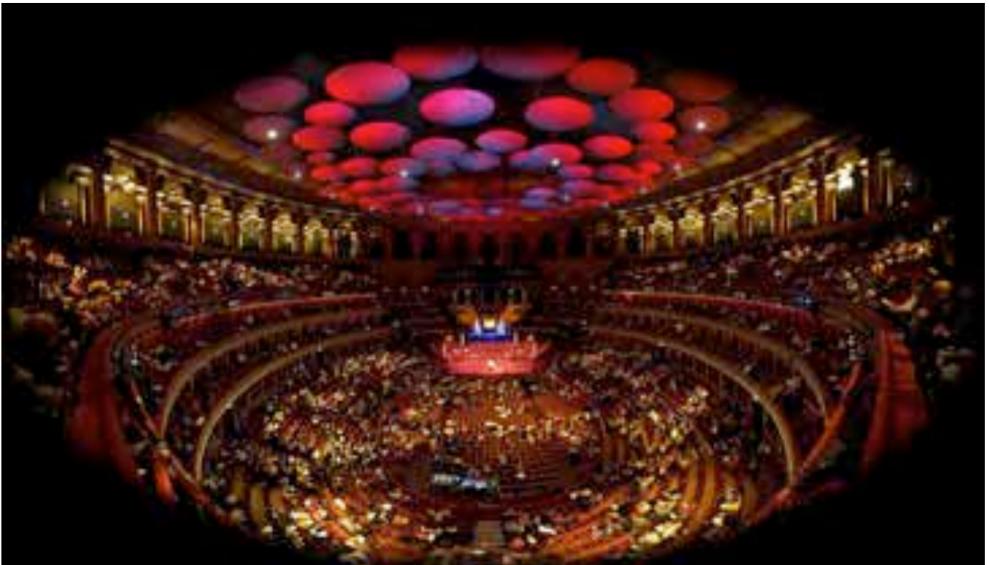
The Royal Albert Hall, London: Large fiberglass acoustic diffusing discs in the roof remove the echo from the Albert Hall. Prior to their installation in 1969, it was said that the hall was the only place where a British composer could be sure of hearing his work twice.
